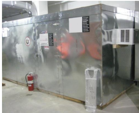
Figure 6-6. Examples of construction shed with sheet metal protection
