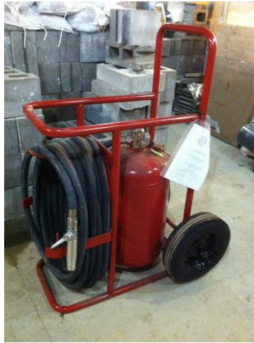
Figure 8-5. Wheeled 40 lb. Fire Extinguisher
