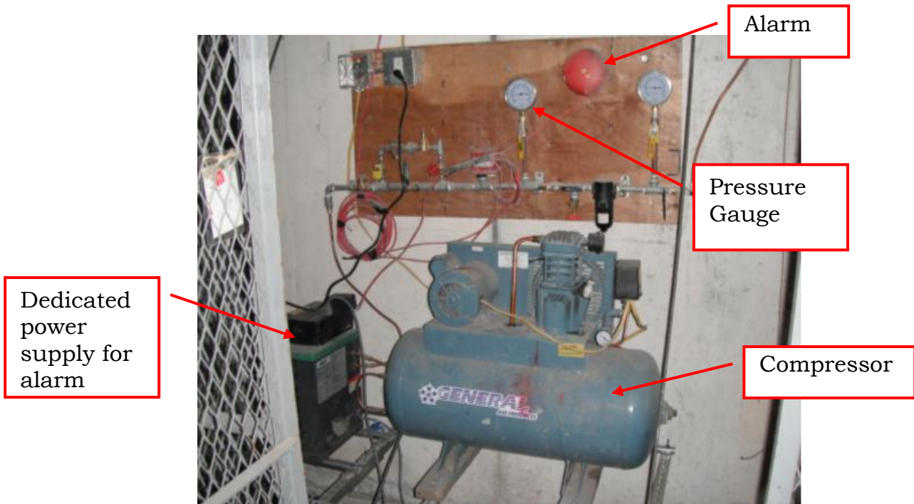
Figure 4-17. Examples of a Standpipe Compressor/Alarm Configuration
