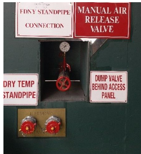
Figure 4-3. Air Pressurized Standpipe System
